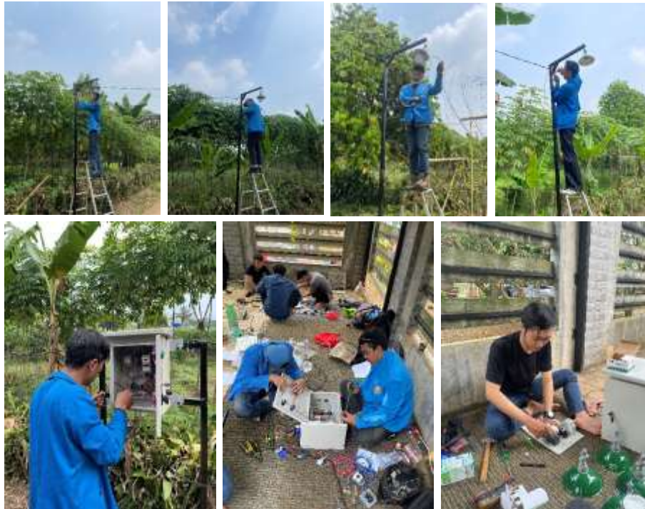
Gambar 5. Proses Instalasi PJU Otomatis Berbasis Sensor LDR
