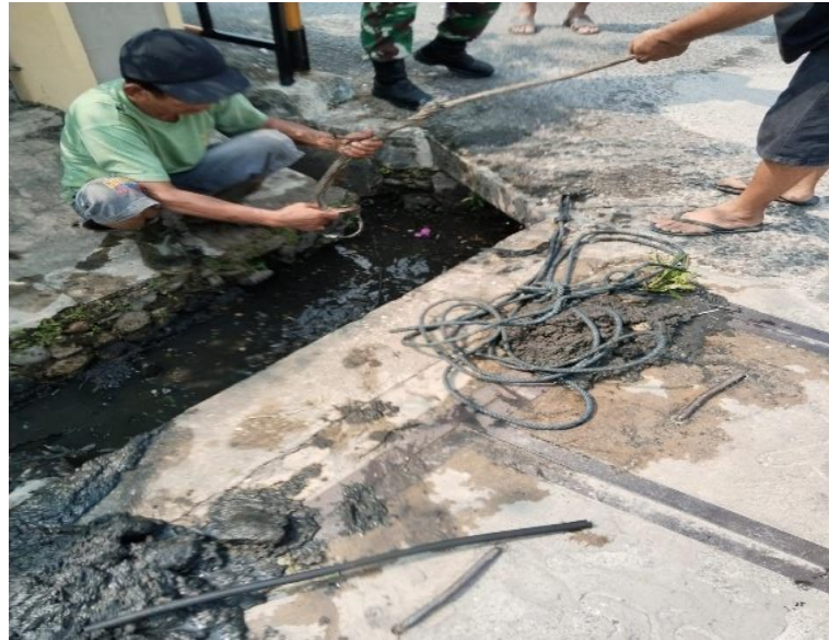
Figure 1. Residents using tools, tyres, steel slings, and vehicles to clean a blocked drainage system on Jl. Arjuna.
