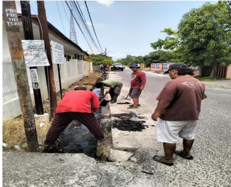
Figure 3. Clearing a blocked drainage channel and removing accumulated waste on Jl. Arjuna
