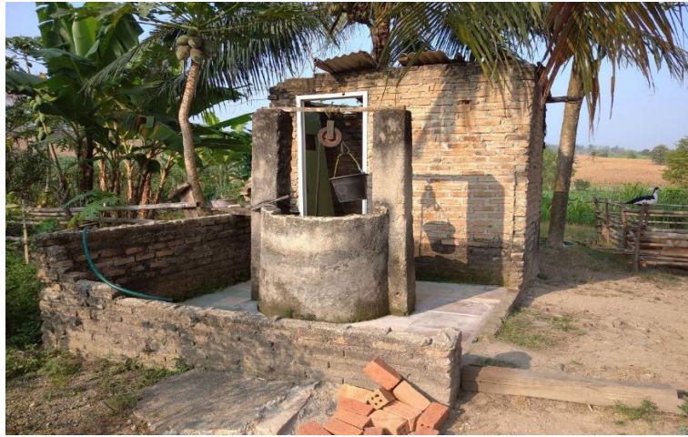
Figure 2. Residents' dug wells, drought during long dry season
