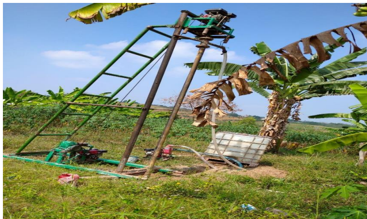
Figure 4. Preparation of borehole installation
