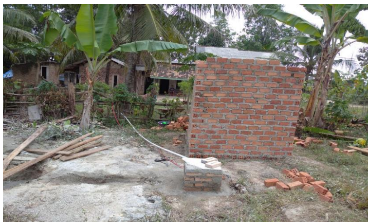
Figure 7. Construction of water towers and water channels to residents' homes
