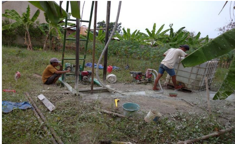
Figure 6. Start drilling the well
