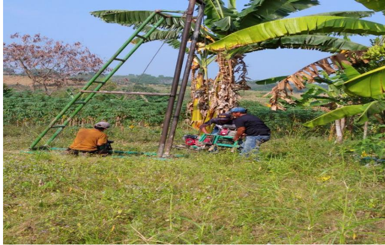
Figure 5. Preparation of machinery and tools for the construction of community boreholes
