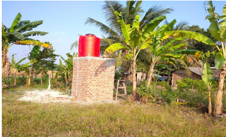
Figure 8. Water installations with boreholes ready to be utilized by residents
