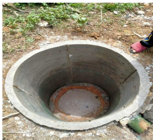
Gambar 10. Dinding Beton Lubang SPAL
