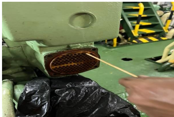
Gambar 2. Proses Pembersihan Fresh Water Cooler
